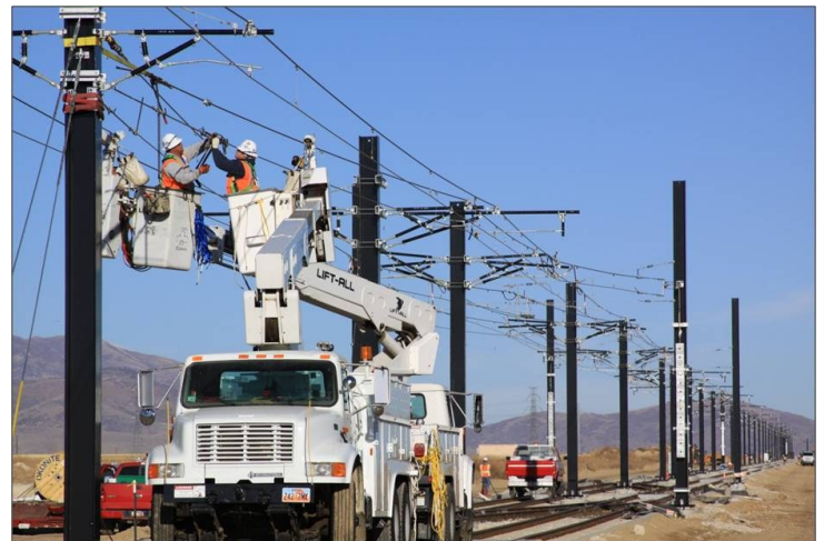
MEC Catenary Workers
