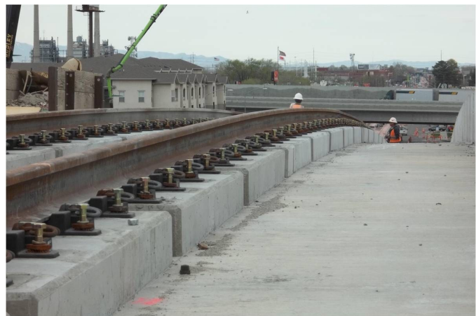
Completed track and plinths on North Temple Viaduct
