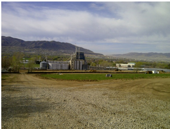
Draper Town Center Park and Ride begins construction
