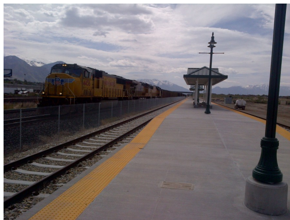
Orem FrontRunner South platform
