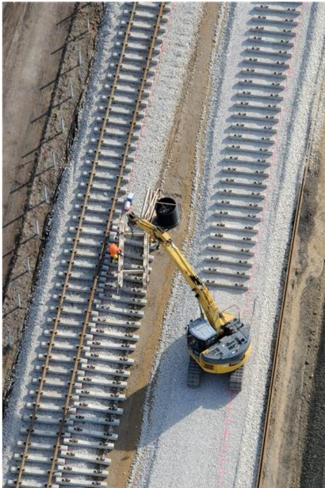
Laying track in Draper
