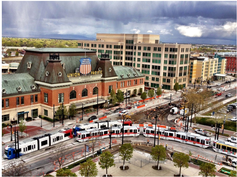
Tie-in track work for Airport Line tracks
