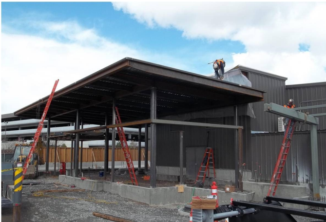
Airport welcome center takes shape
